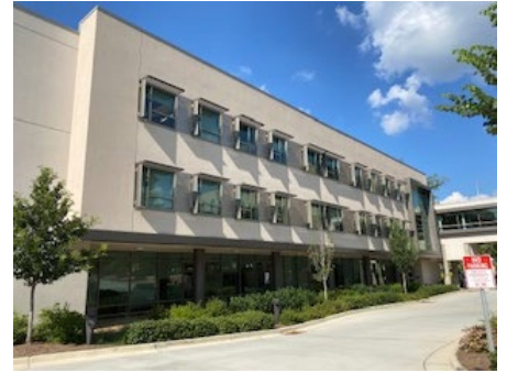
North Building (former education building)
